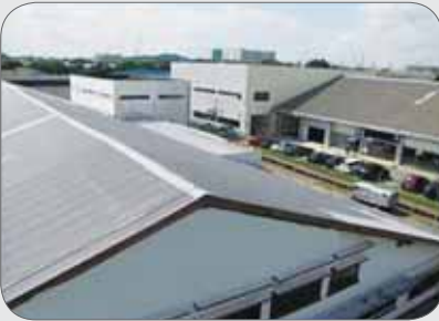
Wide-spanning metal roof of industrial building.
