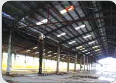
Old industrial building with skylight and roof sheets.
