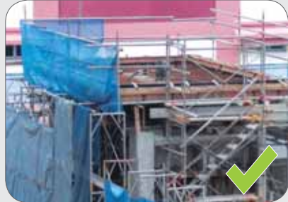
Example of edge protection provided for working on roofs.
