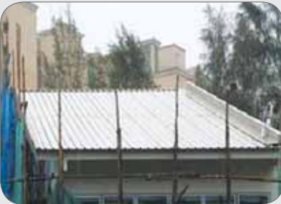
Pitched corrugated metal sheet roof of residential building.
