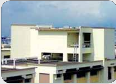
Flat non-fragile roof with low parapet walls.
