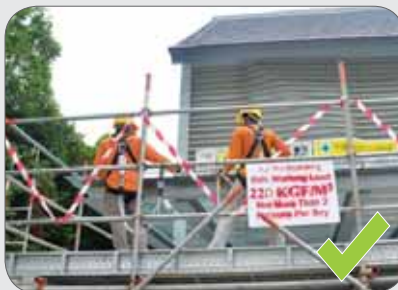
Installation of glass canopy roof with proper access and work platforms.
