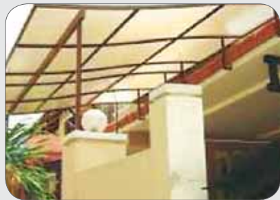
Car porch with polycarbonate roofing.
