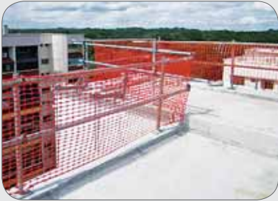
Guardrails erected at edge of flat roof.
