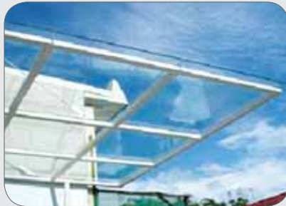
Glass canopy roof of car porch.
