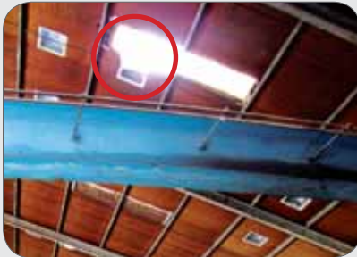
Example of skylight on factory roof.
