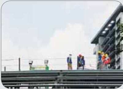
Guardrails erected on roof surface.
