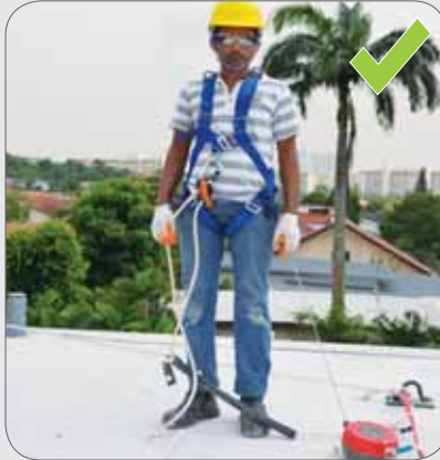
Adequate anchorage and safety harnesses are provided for working on roofs.
