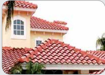
Pitched tiled roof.
